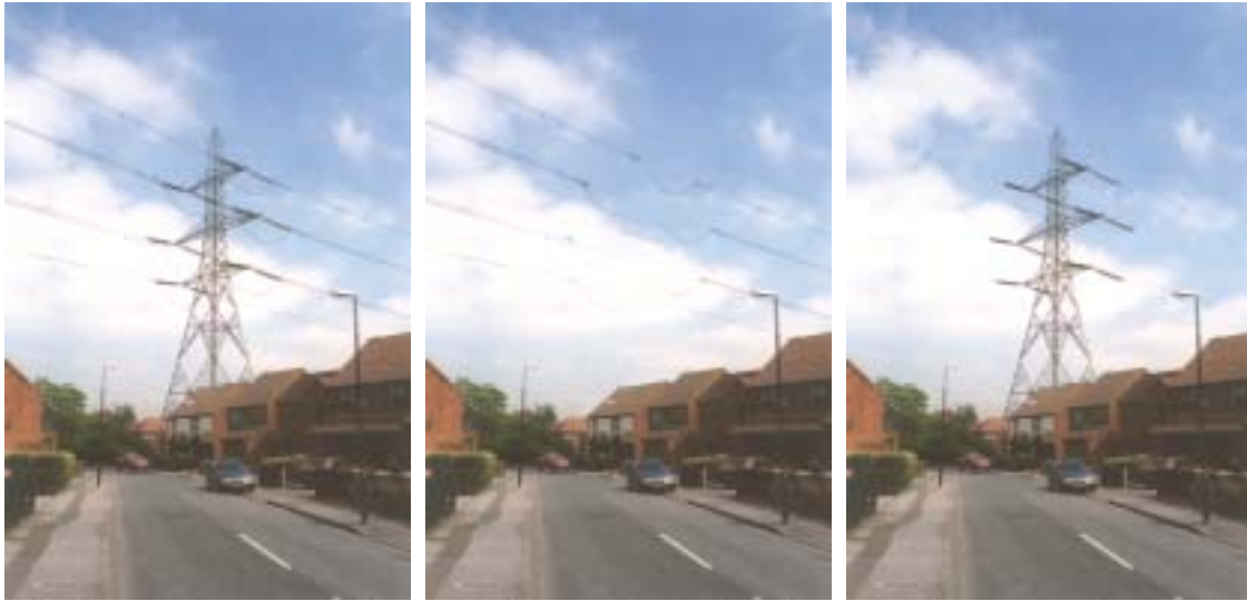
Pylons and lines.
