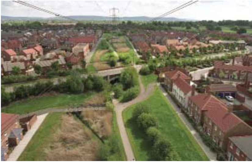
Fairford Leys, Aylesbury. An example of successful integration between development and overhead lines.
